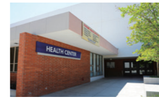
Health Center at Latsia, Cyprus, AHU
