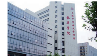
Longhua Hospital, Shanghai, China, AHU
