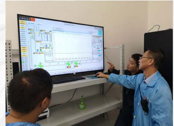
Centralized control system
