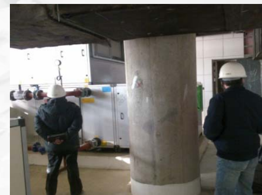
▶ Onsite Picture: AHU Commissioning
