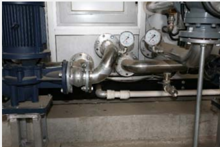
Operation Display of Double Pressure Gauge
