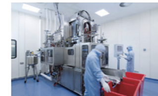
International Pharmaceutical Factory, Cambodia, AHU
